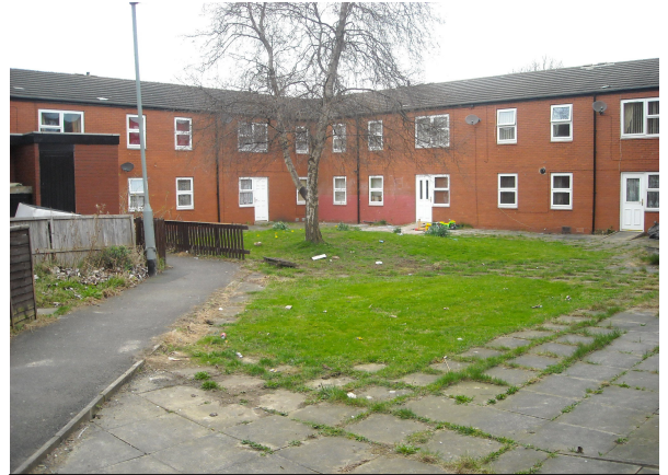
Courtyard allowing access to rear of properties
